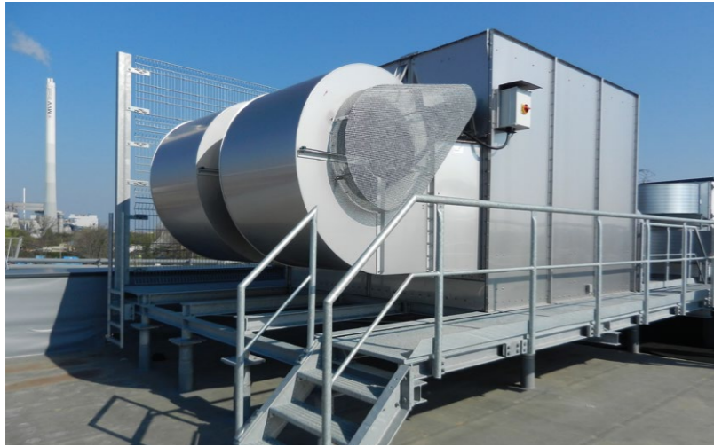
New testing facility - cooling tower
