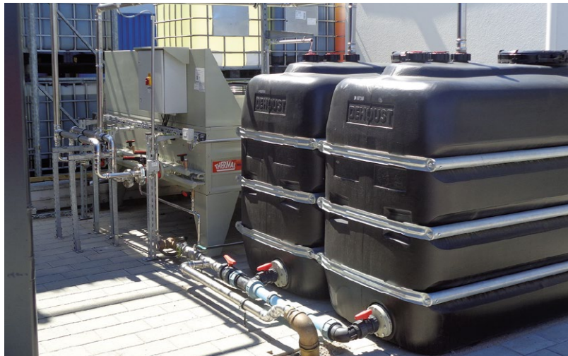
Cold condensate collection with chiller
